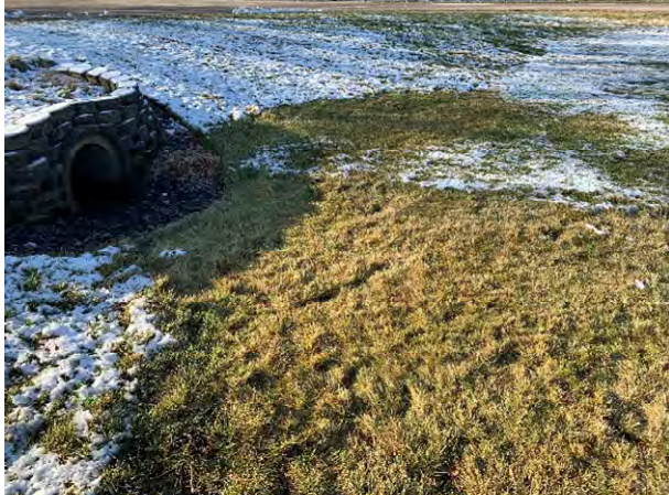
29 Gundalow - 1 (Drainage Area)
