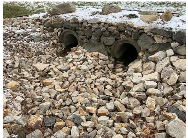
64 Gundalow - 2 (Drainage Course)
