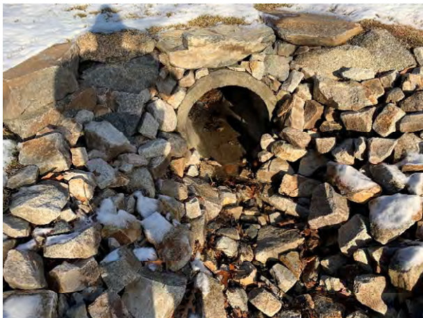
64 Gundalow - 1 (Drainage Course)
