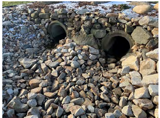
64 Gundalow - 2 (Drainage Course)
