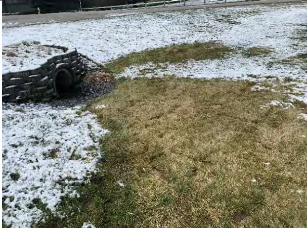
29 Gundalow - 1 (Drainage Area)
